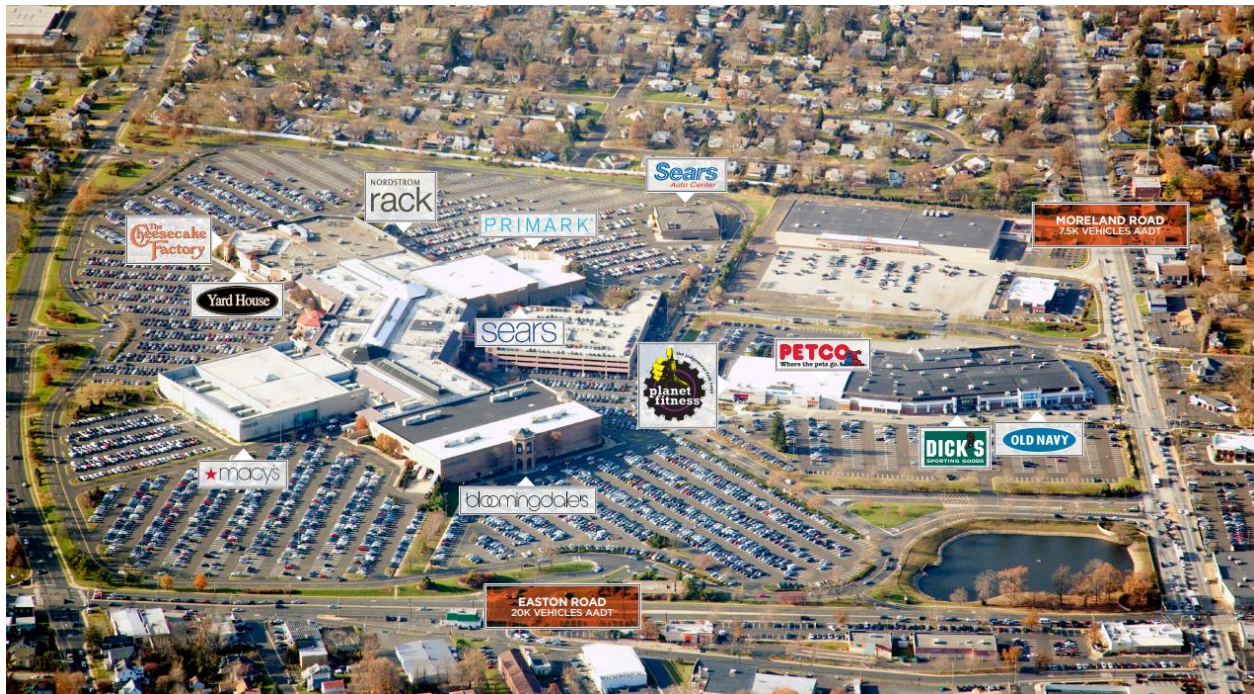
Figure 1: Willow Grove Park Mall Site
